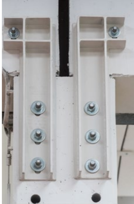
Examples of beam-pillar constraint systems
