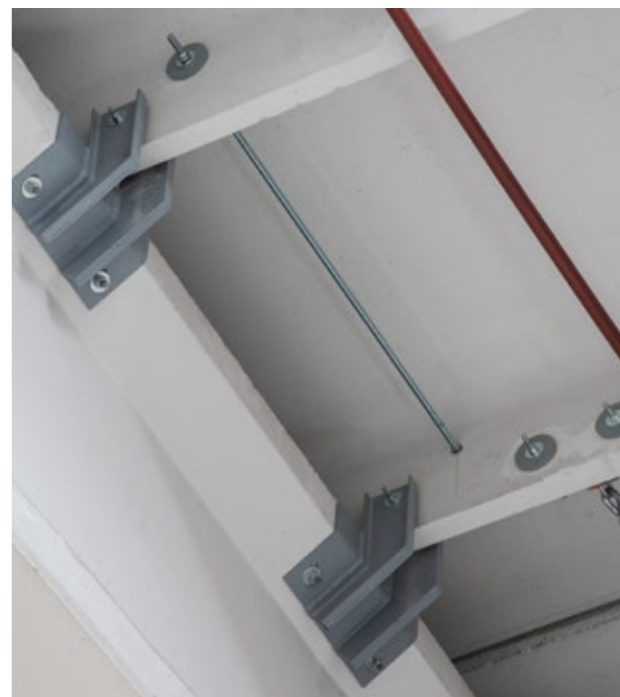
Examples of roof-beam constraint systems
